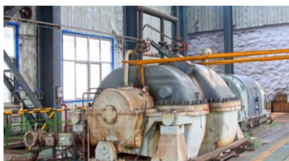
Installation of Top Pressure Recovery Turbines (TRT's) at Blast Furnaces
